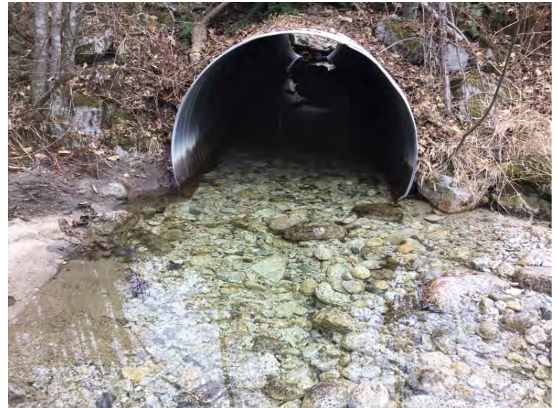
Outlet at high chain culvert
