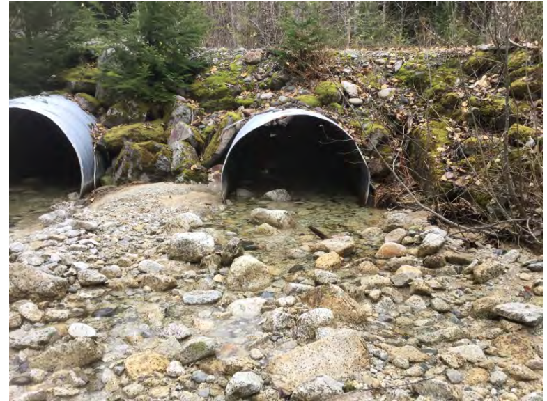
Outlet cover of low chain culvert
