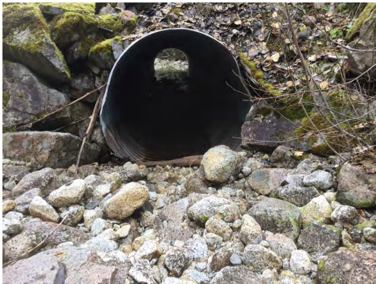
Inlet of high chain culvert
