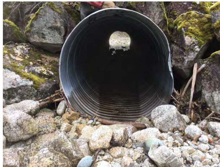
Inlet of middle culvert
