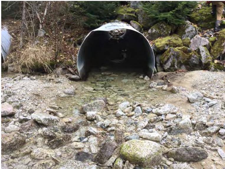
Outlet cover at middle culvert
