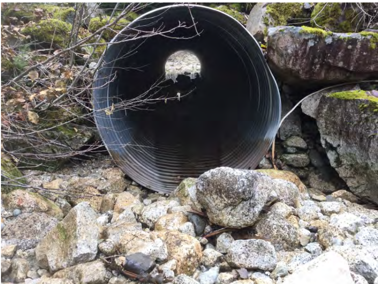
Inlet of low chain culvert
